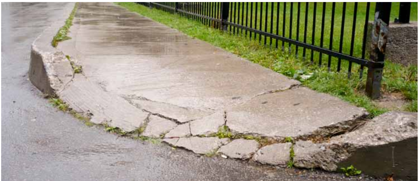
Missing and broken curb cuts in St James Town make sidewalks inaccessible to people with chairs and strollers
